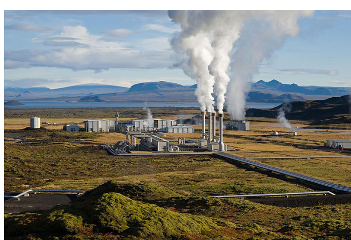
Figure 4: Nesjavellir geothermal power plant, Iceland (Gretar Ivarsson, 2006)
